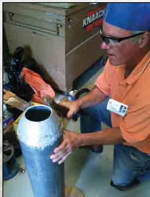
Retired Brother John Murray preparing a lead joint sleeve, in 2017, for a replacement splice at NIH and teaching the younger guys how it was done "old school style"
