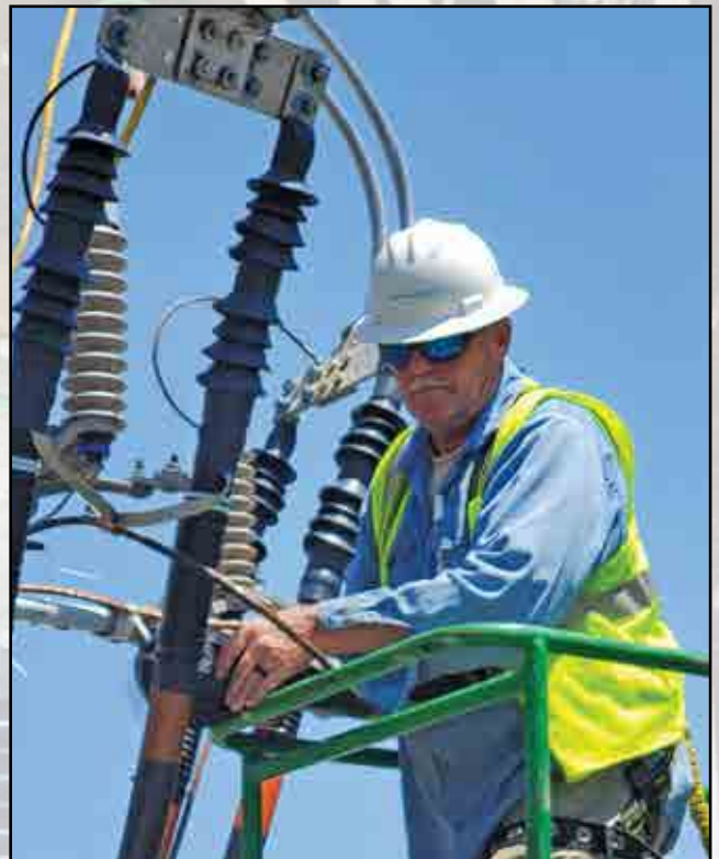
John Honigsberg, Jr., project manager of the Medium Voltage Cable Division, Installing Terminations on 35kv 1 million kcmil cable from a lift in Northern VA at a data facility in 2021
